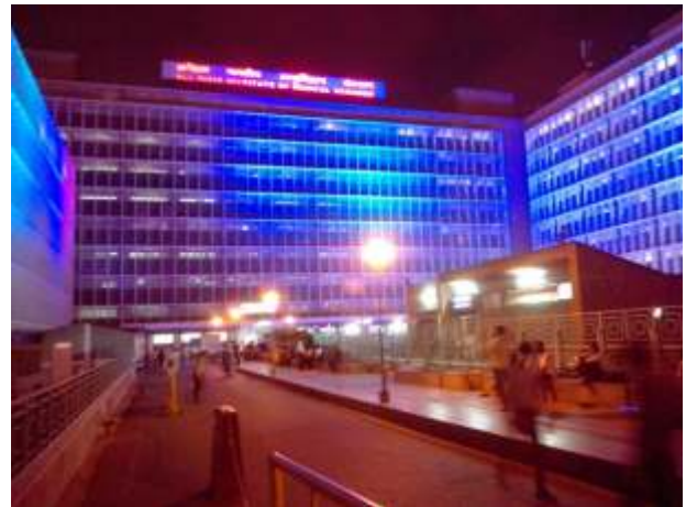
Fig. 2 : The building of AIIMS, New Delhi being lit blue on 30 Apr 2015 to commemorate Autism Day.
